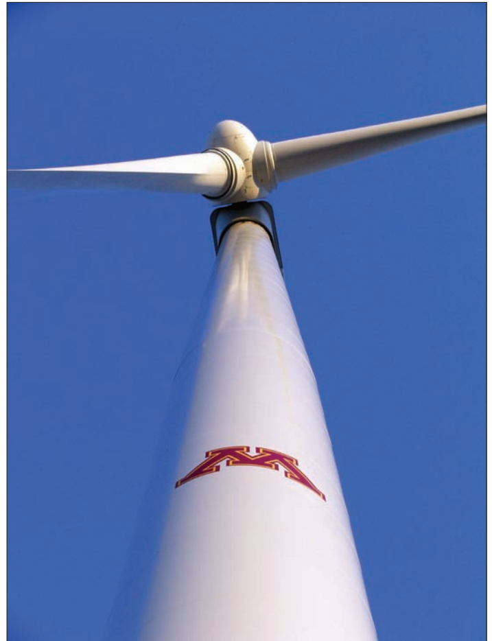
The University of Minnesota Morris is investing in wind power and local biomass.
