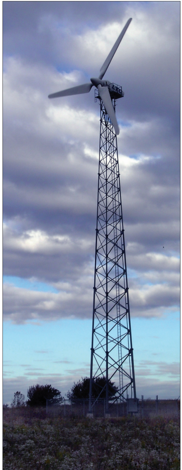
Lakeshore Technical College, Cleveland, Wisconsin.
